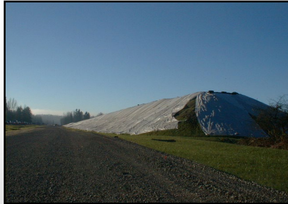
Poor protection of stockpiles
